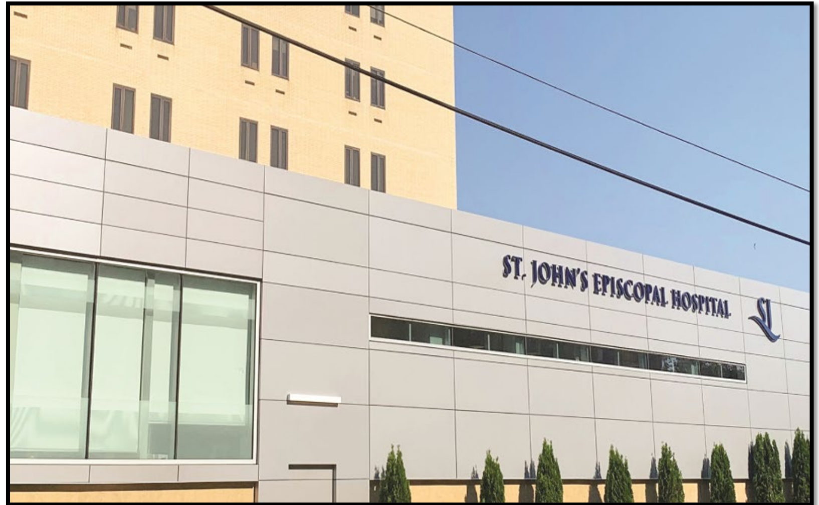
St. John's Episcopal Hospital Campus, Far Rockaway, NY
